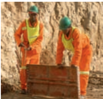
ROAD CONSTRUCTION, HOSPITAL BEND
