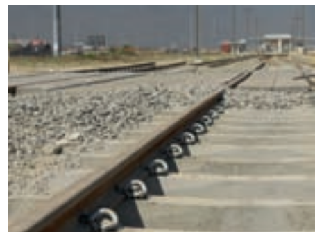
URBAN RENEWAL PROGRAMME RAIL UPGRADE, KHAYELITSHA
