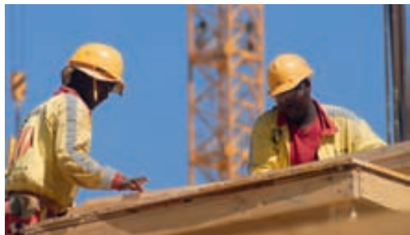
CONSTRUCTION OF GREEN POINT STADIUM
