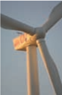
DARLING WIND FARM
